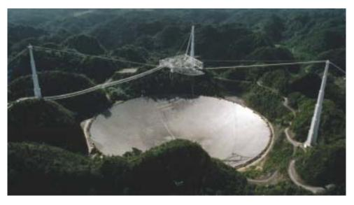
**Figure 3.11** Because the wavelengths of radio waves are so large, the antenna of a radio telescope must be large. This radio telescope in Arecibo, Puerto Rico, has a diameter of more than 300 m. That's almost the length of three football fields laid end to end.
